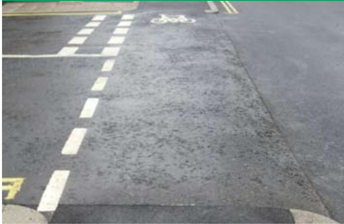
The recent improvements to the Old Shoreham Road in Brighton include a standard detail for providing enhanced cycle priority when tracks run past minor side streets.
